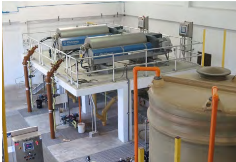
High-solids dewatering centrifuges installed at the City of Sunrise Sawgrass WWTP
