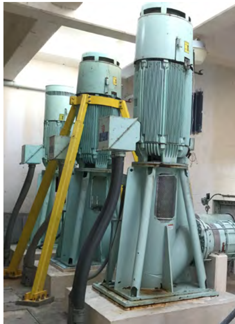
Injection well pumps
