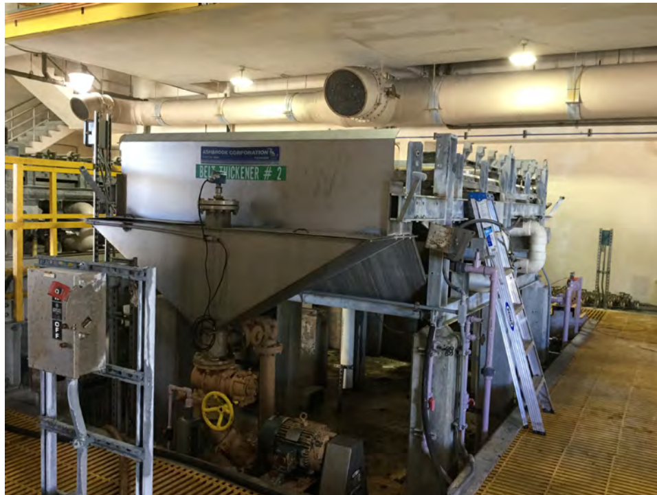
Existing gravity belt thickener at the Miramar WWRF
