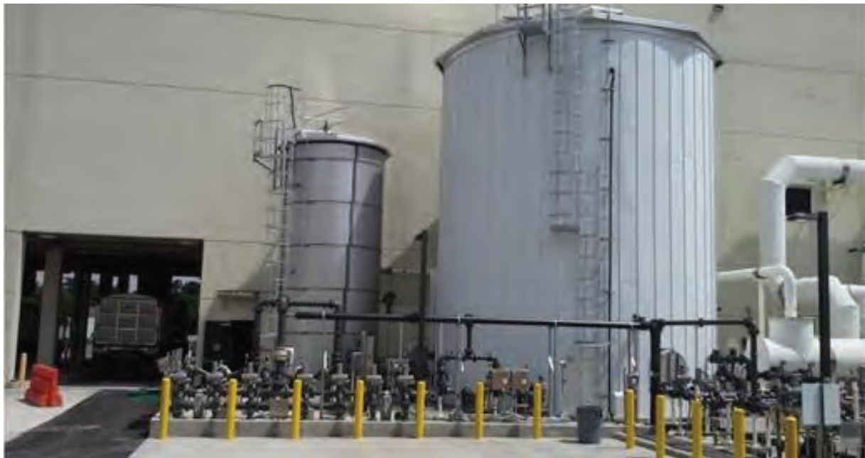
Above: North Regional WWTP Installed FOG Receiving and Dosing System. The biogas collection and treatment, CHP facilities and the FOG receiving station started operation at the end of 2015 and continues to operate today, saving Broward County over $1.5 million annually in electricity costs.
