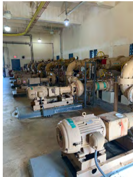
Return activated sludge pumps at the Miramar WWRF
