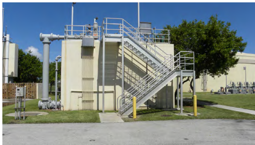
Dynasand filters with EcoWash
