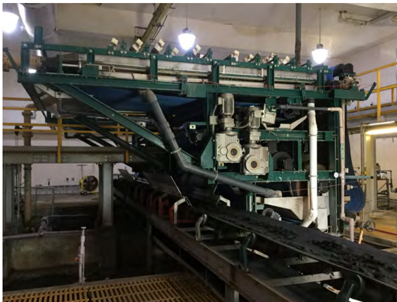
Existing belt filter press at the Miramar WWRF
