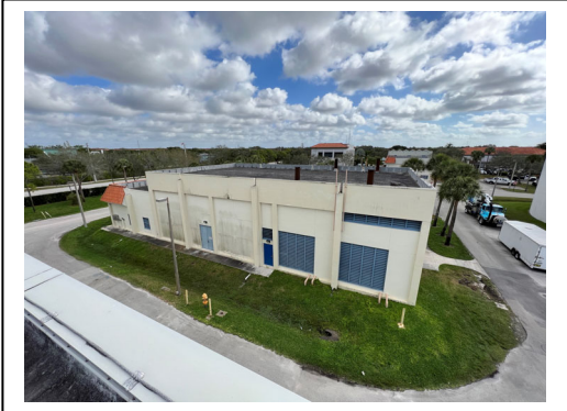
Miramar – Wastewater Treatment Plant
