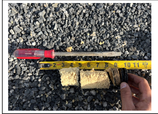
Roof A – High Core Sample
