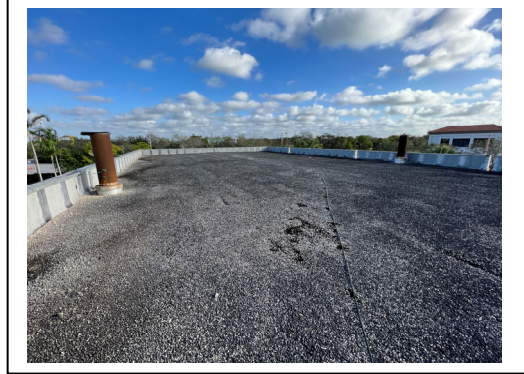
Roof A - Overview
