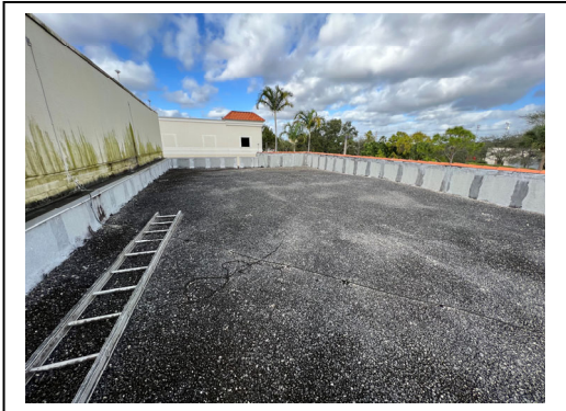
Roof B - Overview
