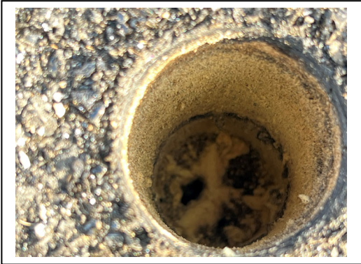
Roof A – High Core Cut
