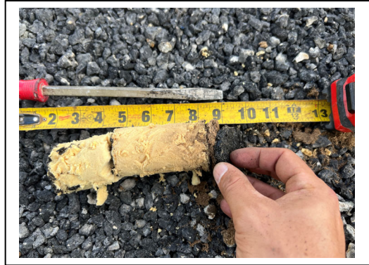
Roof B – High Core Sample
