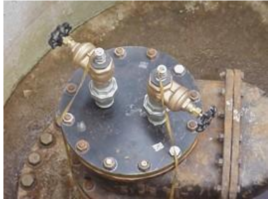
Figure 7: Combination Insertion and Pull Site
