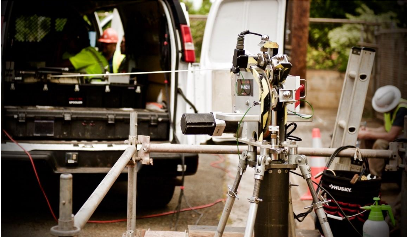
Figure 4: Sahara Insertion Assembly, Winch, and Cable Drum with Continuous Sanitation
