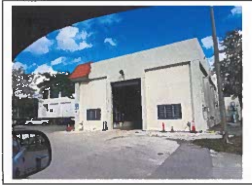
Miramar – Wastewater Treatment Plant
