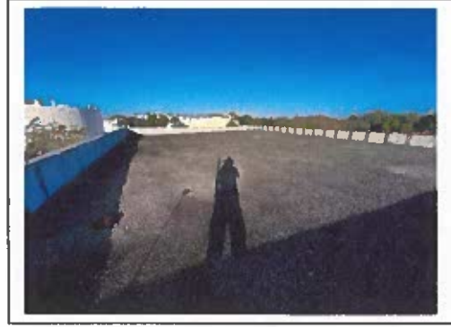
Roof A - Overview
