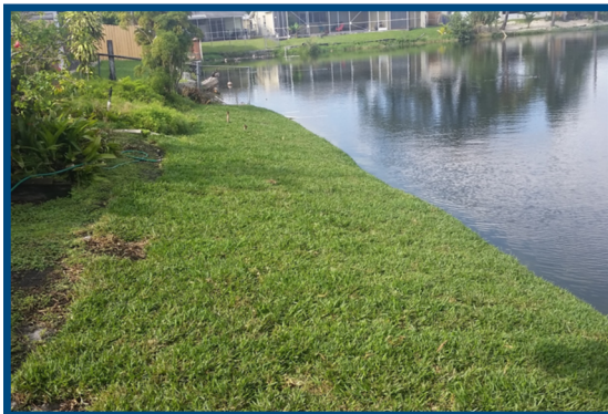
Historic Miramar Canal Improvements
