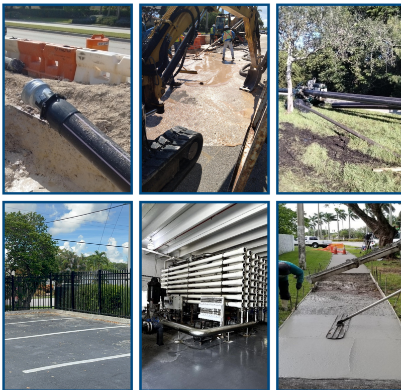
Various Infrastructure Improvements
