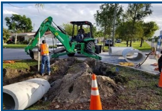
Citywide Embankment Stabilization and Stormwater Management
