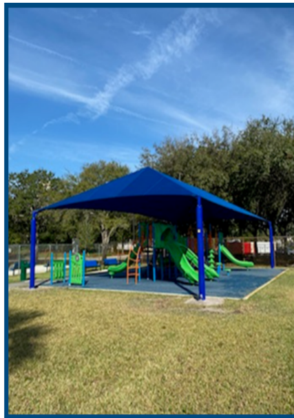
H.D. Perry Park Playground Shade Cover Addition
