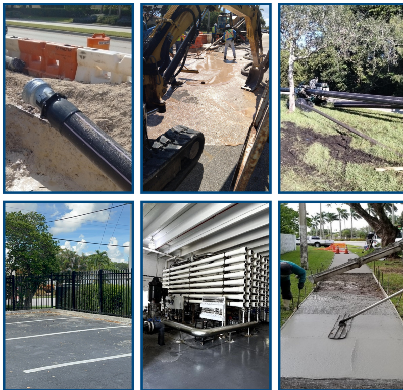
Various Infrastructure Improvements
